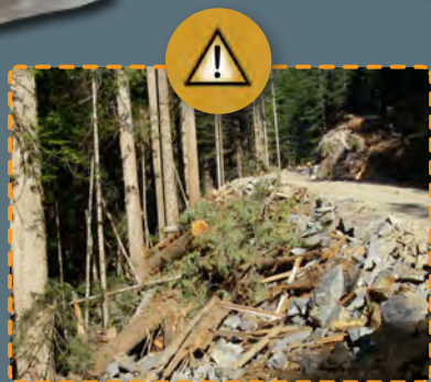
Stumps, boulders and debris hung up in standing timber
