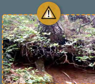
Unstable or undermined trees or stumps
